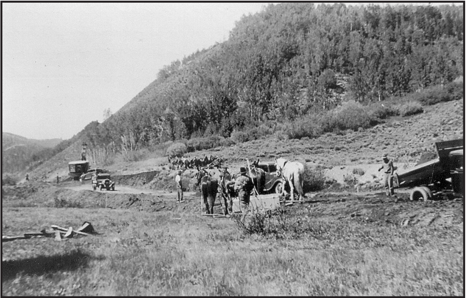
Building the road on Salt Creek
